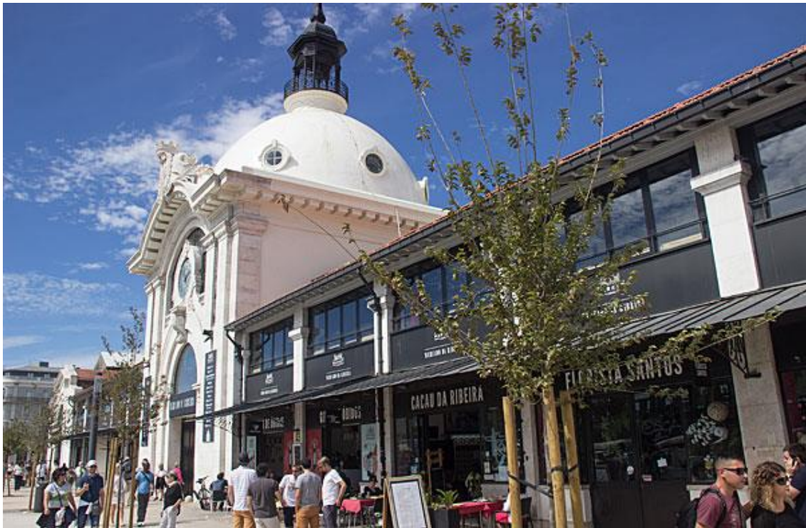
Figura 22 – Fachada do Time Out Market
